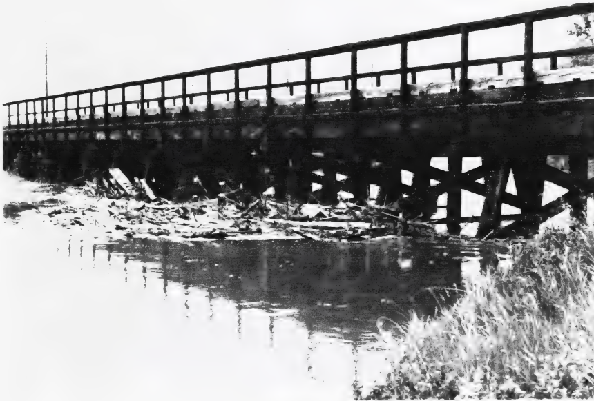
u/s side of bridge HWM VR 83-2 28 June 1983
